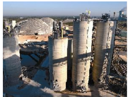
NGS Ash Storage Silos
